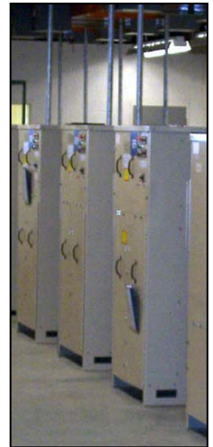
Ferromagnetic Reactor Type, Air Cooled, Comparable to Ferro-resonant Type
