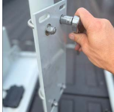
2. Secure the mounting pipe to the mounting plate using supplied u-bolts.
