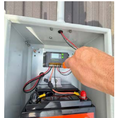
5. Connect the red and black wires to the charge controller.
