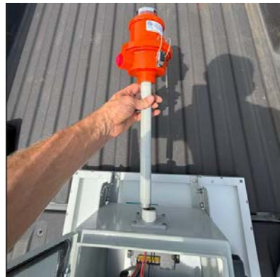
4. Install the Obstruction Light to the enclosure by running the wires through the top hub and then tightening the pipe.
