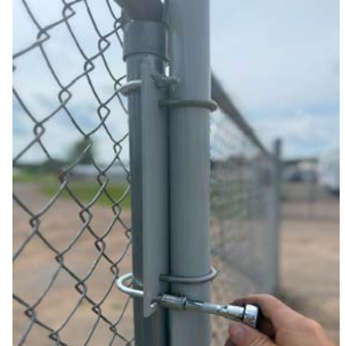
3. Secure the mounting plate to the fence post.
