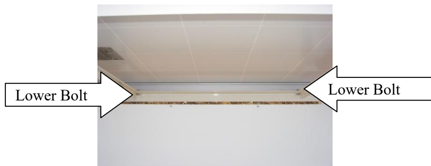
Figure 9. Lower Solar Panel Mounting Bolts
